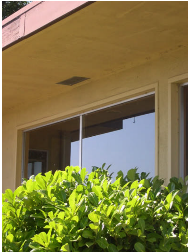
This plant immediately under the a vent (and next to a single pane window) could be a problem if it ignites.
