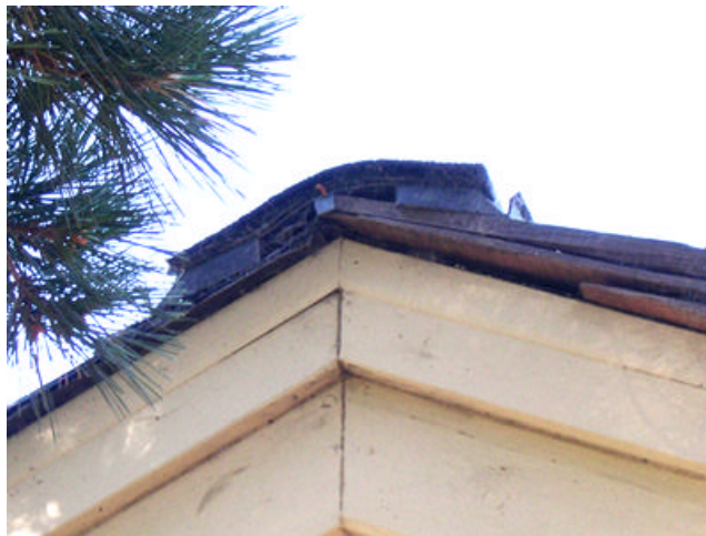
A ridge vent (as seen from the side of the roof) that is found along the entire ridge of the roof. Baffles along the front edges of the vent keep rain from entering and provide for a negative pressure region that helps pull air out of the attic.
