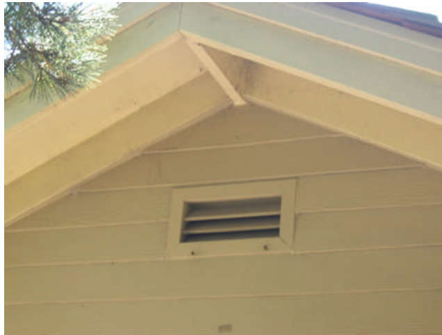
A gable-end vent, usually located just below the ridge of the roof.
