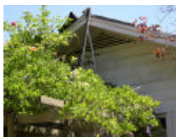
This trellis vegetation could also expose the gable-end vent to embers or flames.
