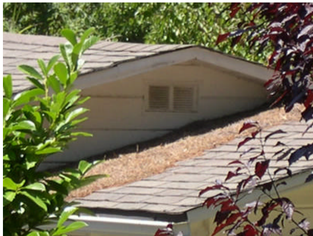
Needles (debris) from near-by pine trees that have accumulated on the lower roof section could easily ignite from embers and subsequently expose the gable-end vent to embers or flames.
